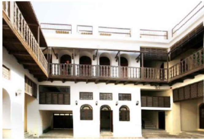
Fig.5. Increasing walls shaded area in Tabib House in Boushehr by using arcades; (Source: Cultural Heritage Organization, Boushehr Province)
