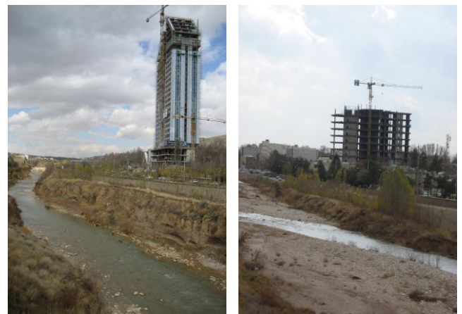
Fig. 2, 3. Effects of construction on the river landscape
