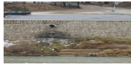
Fig. 8, 9. Effects of pollution (visual & environmental) on the ecology and landscape of the Khoshk River
